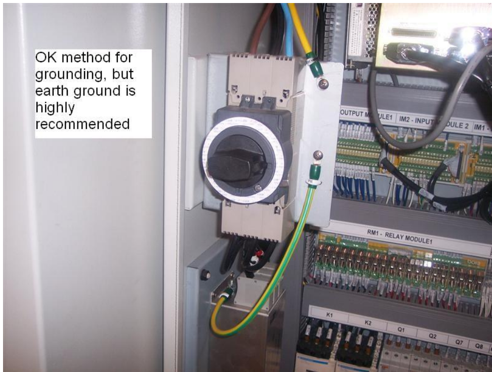
Figure 10 – Alternative method for grounding the LPM
