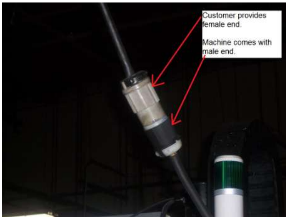
Figure 6 – Power cable example
