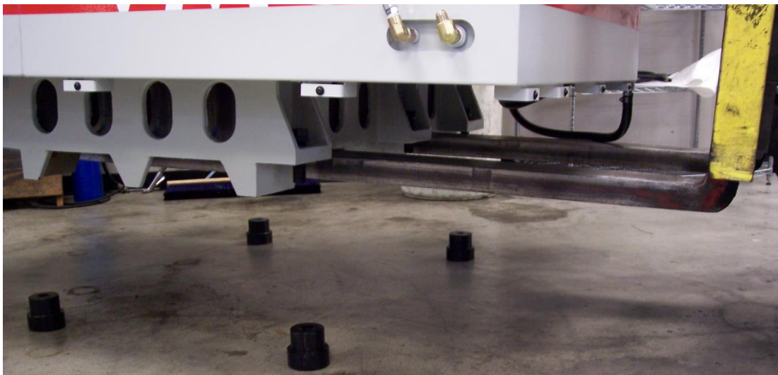
Figure 2.4b - Detail of Fork lift blades set in TMC base and proper set up of Leveling Pads
